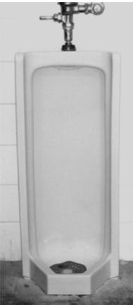
Floor urinals for the most part have been replaced in contemporary construction by wall mounted urinals. Wall mounted urinals are preferred by most building owners because, like wall mounted toilets, they leave the floor unobstructed and therefore easier to clean. Whether they
